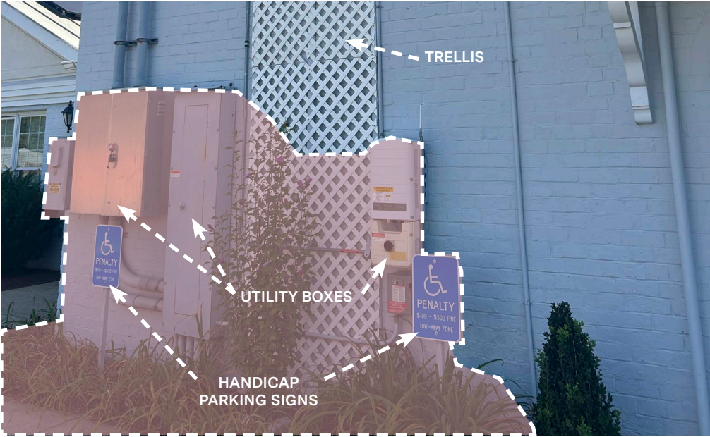
Solar utility boxes. Opportunity to enhance screening and provide educational signage about solar energy. Recommended increase of height of handicap parking signs to meet code.
